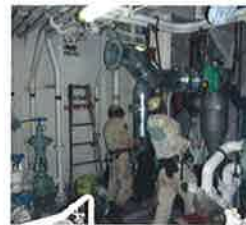
Works for installation
